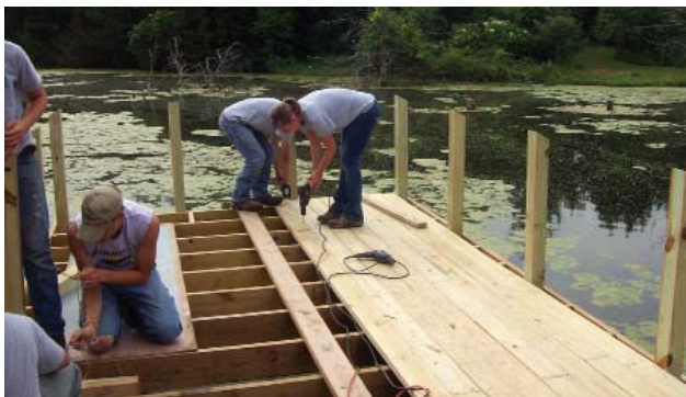
Installing the deck on the Heron Hideaway Pond fishing dock.
