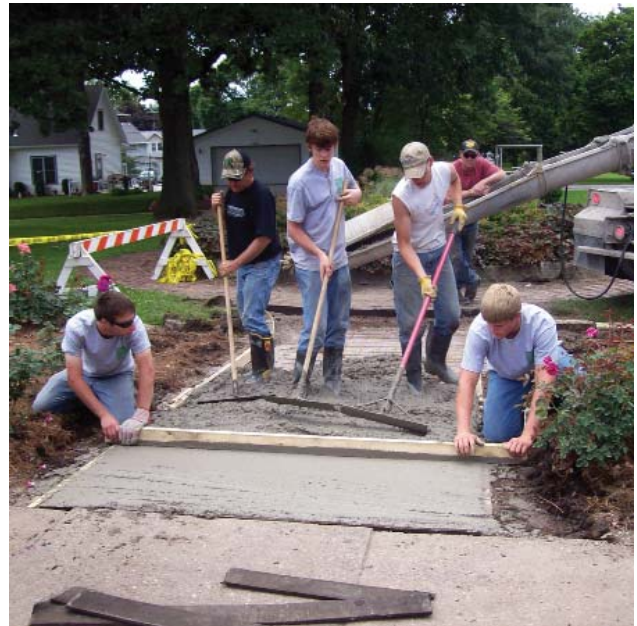
Pouring a sidewalk at the Weed Park Rose Garden
